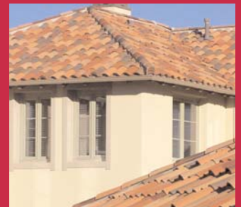
“Class-A” roofing and dual pane windows
